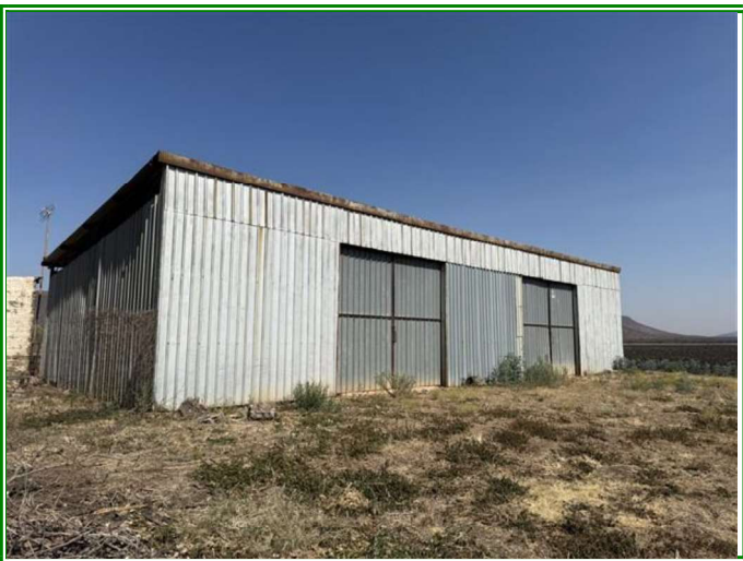
Corrugated Shed (F) (Northern View)
