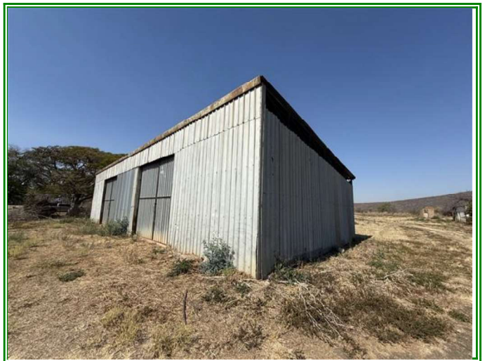
Corrugated Shed (F) (Western View)
