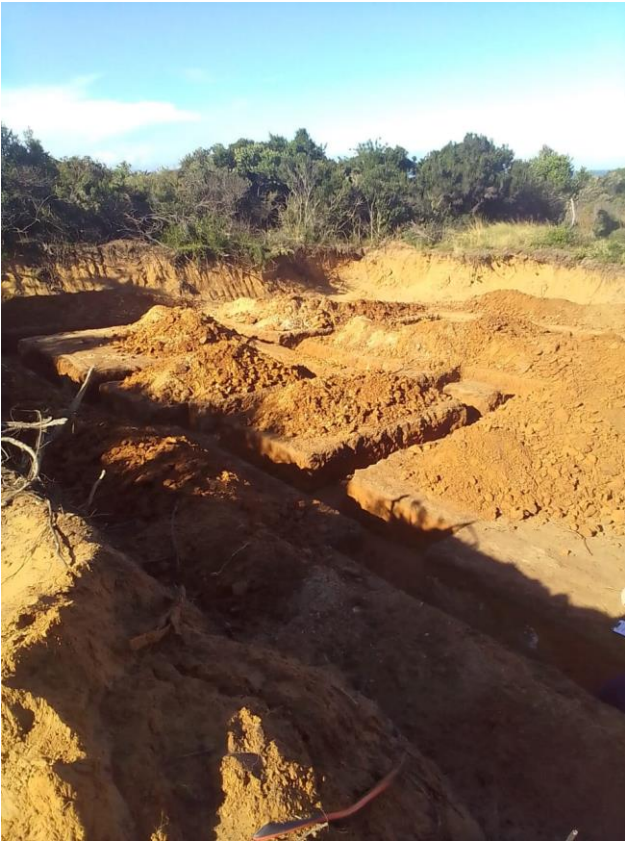
Plate 1: Foundation excavations in firm sandy soil
