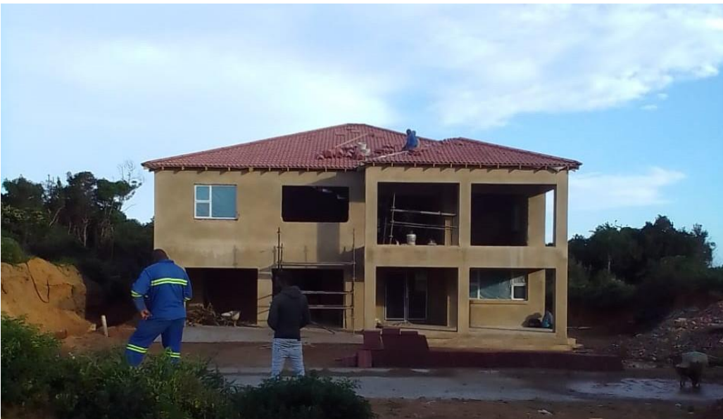
Plate 10: Installation of roof covering
