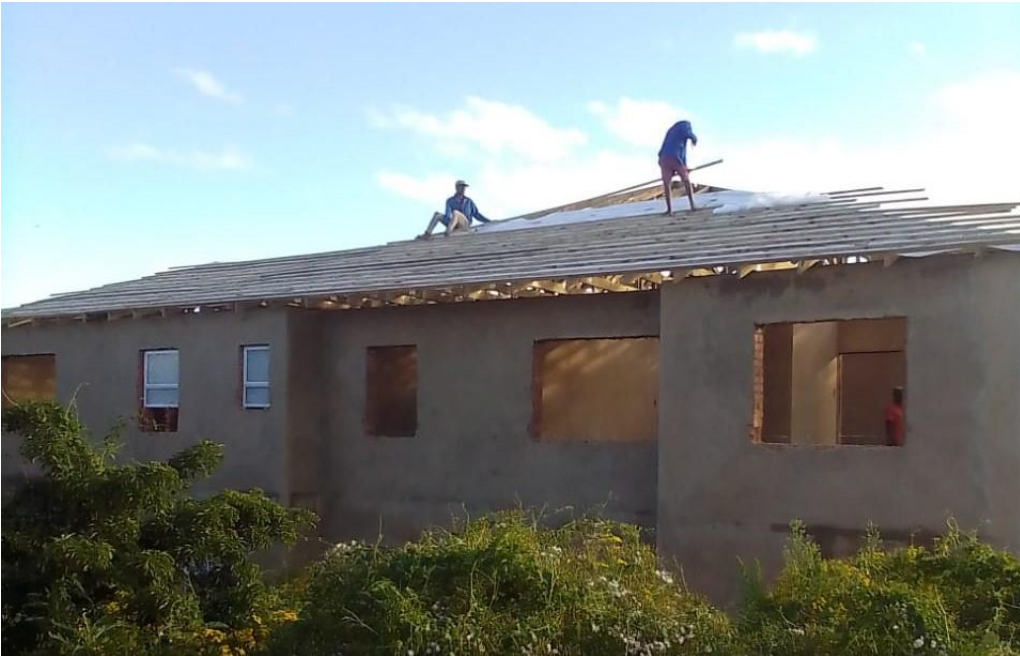
Plate 9: Prefabricated roof installation
