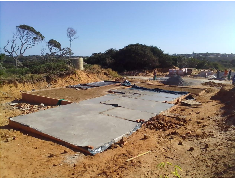
Plate 4: Underfloor compaction and Casting the groundfloor slab
