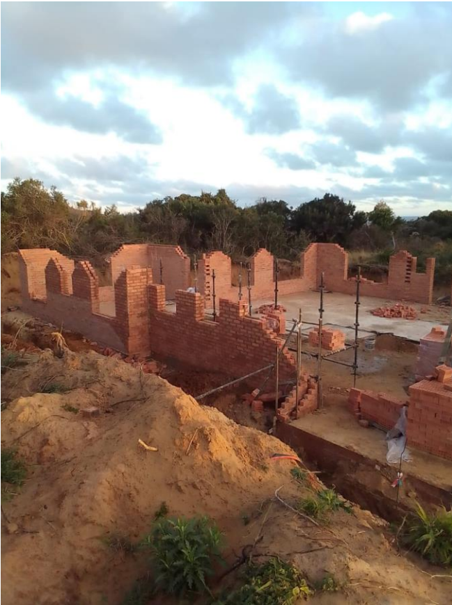
Plate 5: Groundfloor brickwork in progress
