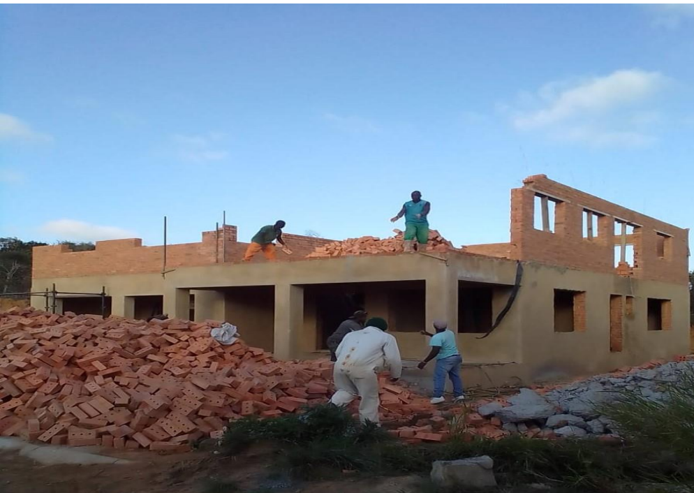
Plate 8: First floor brickwork in progress
