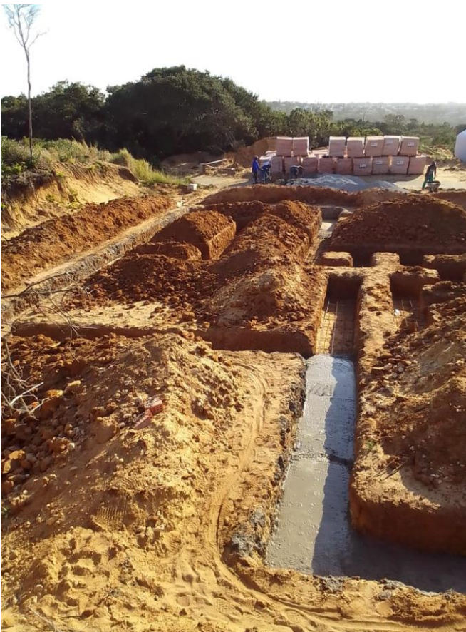
Plate 2: Casting the reinforced concrete footings
