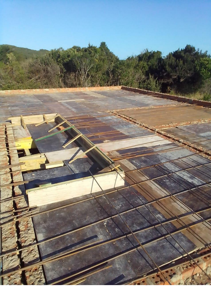
Plate 7: Formwork and commencement of first floor slab reinforcement fixing
