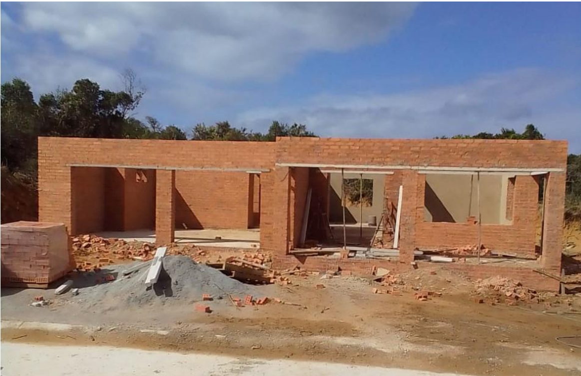
Plate 6: Groundfloor brickwork complete
