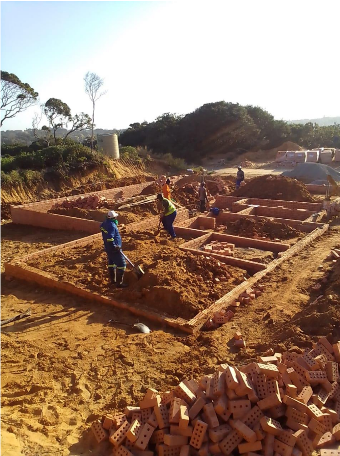
Plate 3: Foundation Brickwork
