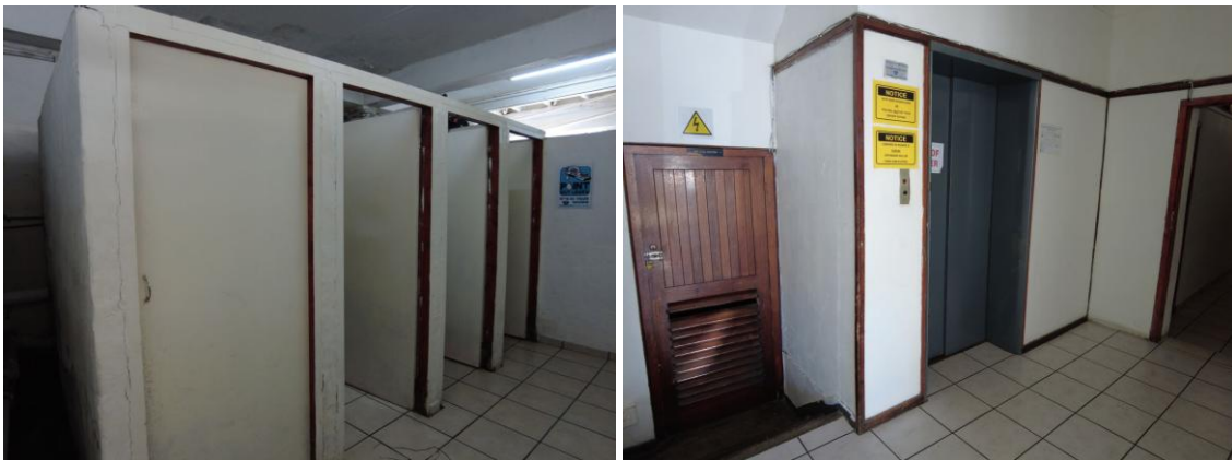
Ground floor communal showers and lift
