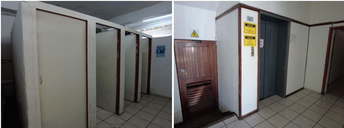
Ground floor communal showers and lift
