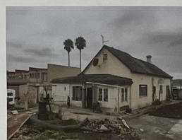
REAR SIDE OF THE BUILDING
